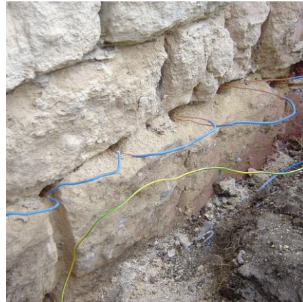
Figure 4 : Treatment of damp walls with electro-osmosis; (left) Water ascends in the capillaries of the positive pole (the ground) towards the negative pole (the wall), thus inflicting damage; (right) inserting electrodes into the wall (copper, positive pole) and in the ground (iron, negative pole) inverts the natural wall / ground polarity, and the passage of water changes direction. Some mortar is then injected by electrophoresis to block the capillaries (photo credits Sté Sofrelop).
